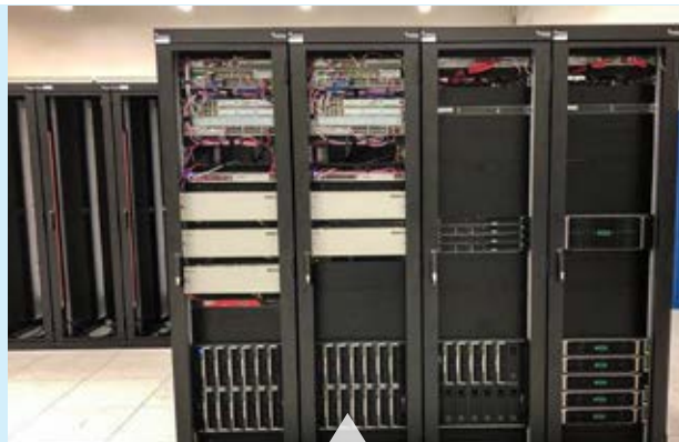
Server room build in progress
