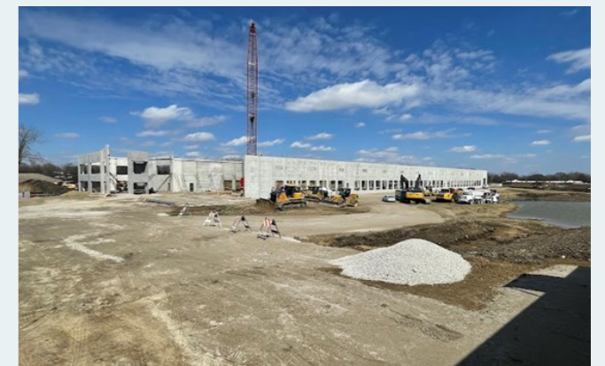
Quick progress has been made as tilt slab construction commences in West Chicago
