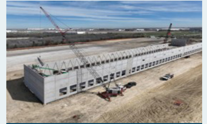
Quick progress as tilt slab construction commences at Haslet, Texas
