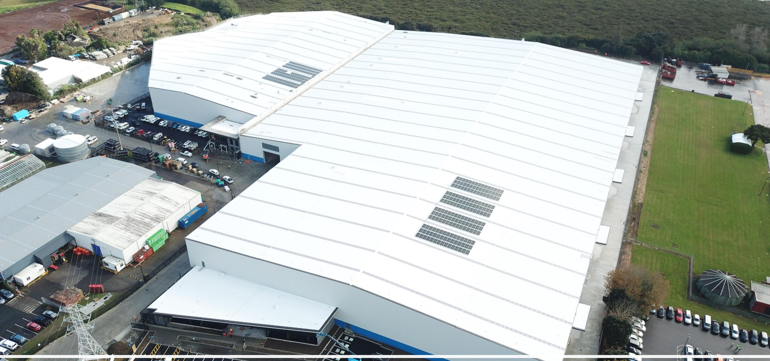
FAVONA, Auckland – Completed
